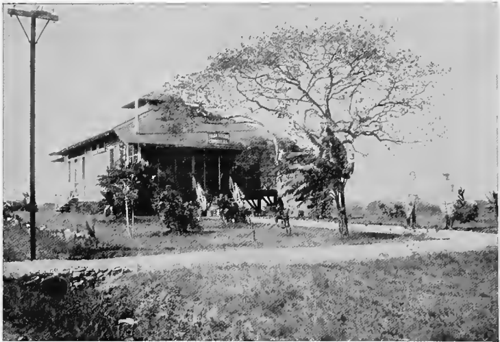
Corozal Police Station
